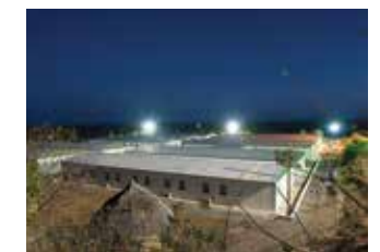
Remote Site/Camp Solutions
